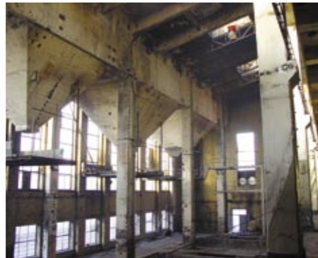
The former power station will become a cultural and sports centre hosting theatre, music, concerts, dance and education.
